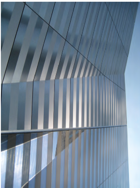
PROJECT: NATIONAL SEPTEMBER 11 MEMORIAL MUSEUM PAVILION ADDRESS: GROUND ZERO, NEW YORK, USA CLIENT: NATIONAL SEPTEMBER 11 MEMORIAL MUSEUM & MEMORIAL ARCHITECT: SNØHETTA LANDSCAPE ARCHITECT: PETER WALKER AND PARTNERS PHOTO: THE ARCHITECT
